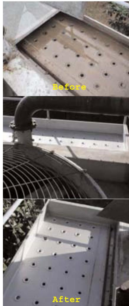
used Cortec's high performance, moisture cure urethane coating - VpCI-396 - on the distribution deck of the cooling tower. The pictures shown are before, and then after, one year of performance.
